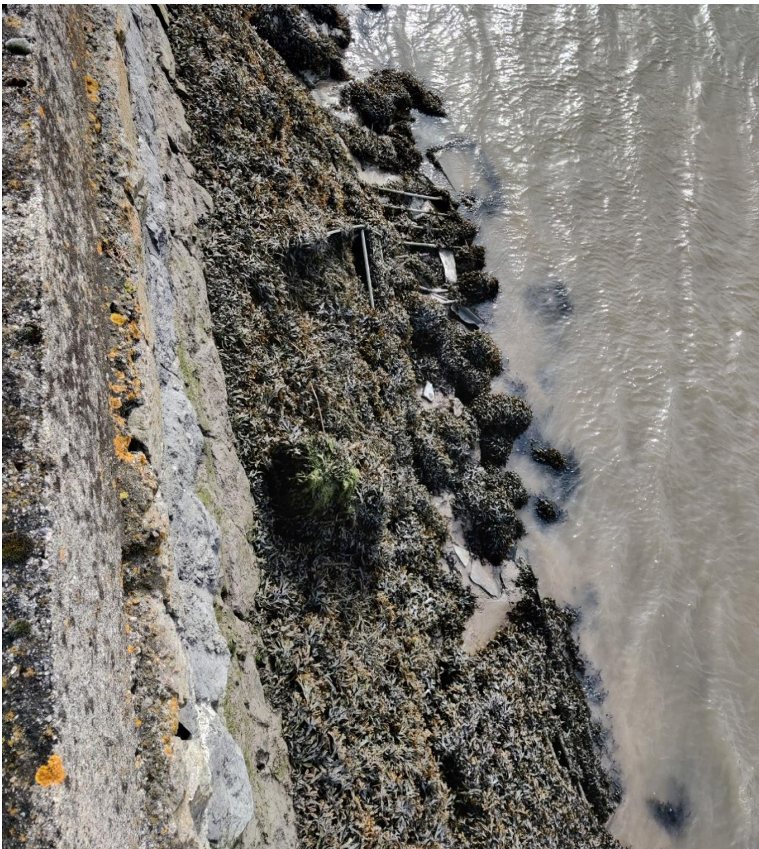
Plate 2.14 Existing quay wall surface with Fucus spp. community.
