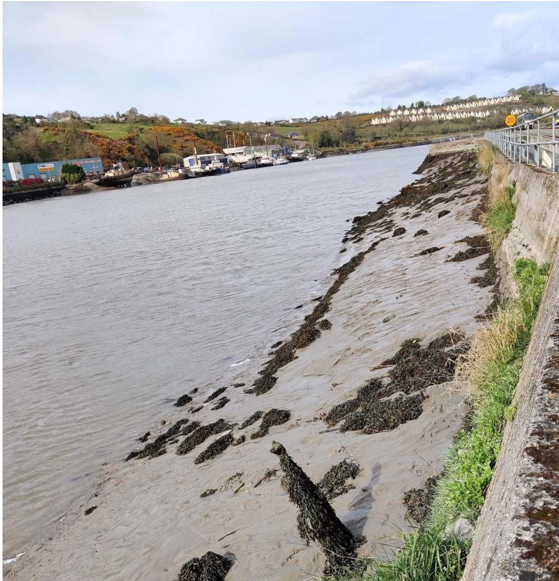
Plate 2.16 'Mud shores' at the western end of the proposed extent of the new riverside flood defence wall.
