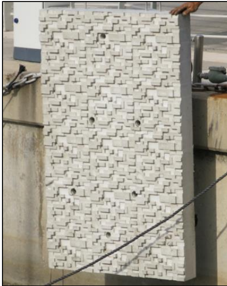
a) Installation of an eco-seawall
