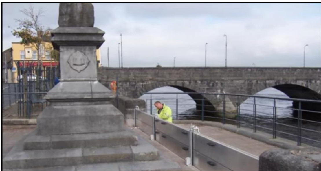
Plate 2.6 Demountable Flood Barriers at Clancy Strand, Limerick (Source: www.floodgateireland.com )
